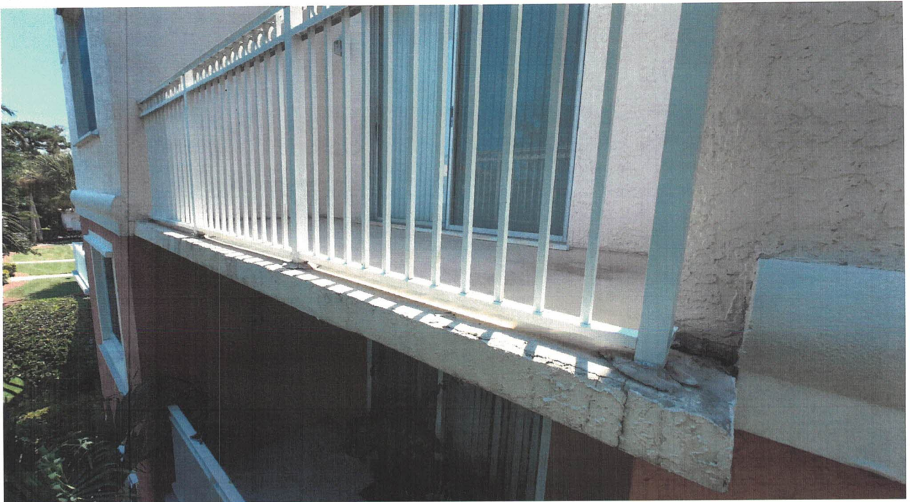
Unit 8310 - Spalling at corner post
