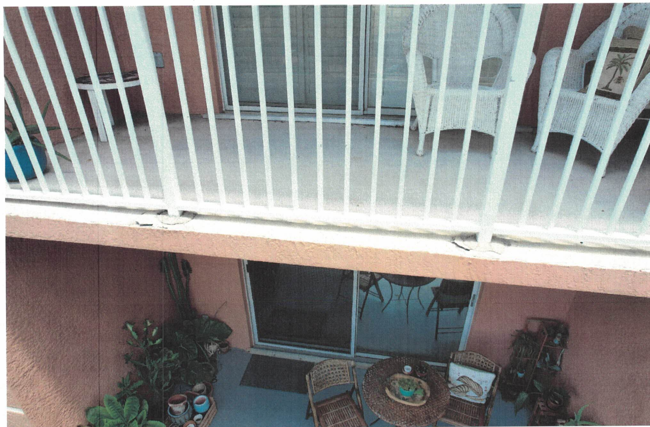
Unit 4204 - Light spalling at base of posts
