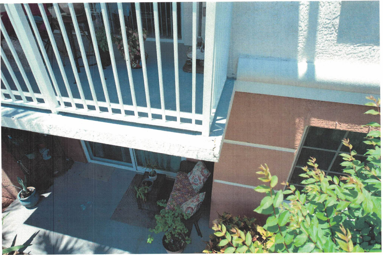
Unit 6202 - Spalling at corner post
