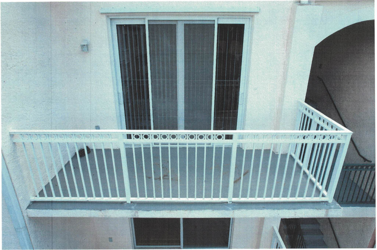
Unit 3310 - Light spalling at base of posts
