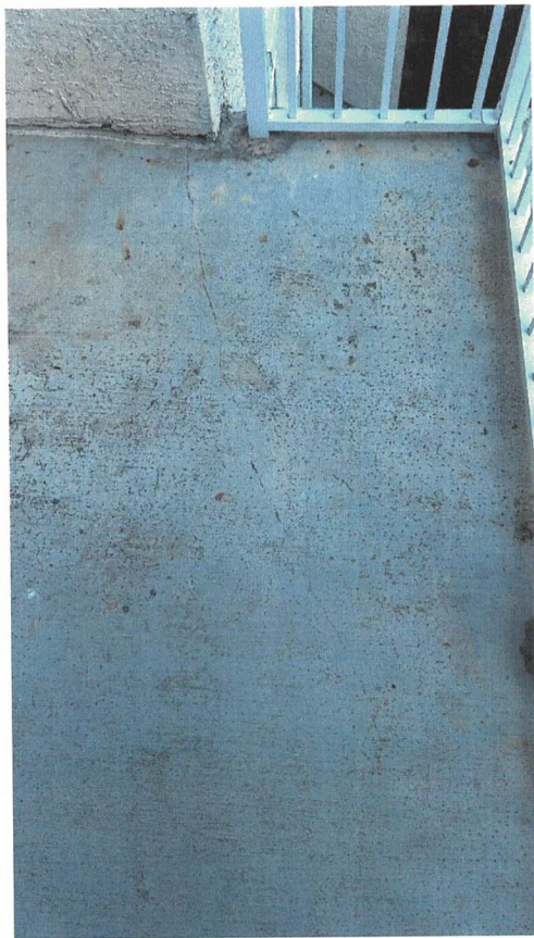
Unit 6308 - Light cracks in balcony slab
