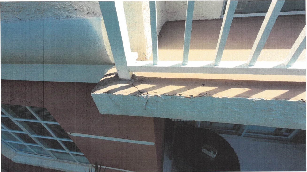
Unit 1212 - Spalling at corner post
