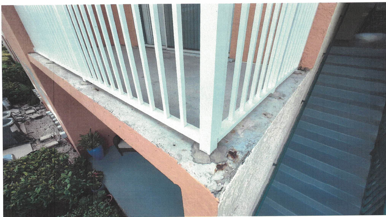
Unit 9206 - Exposed rebar
