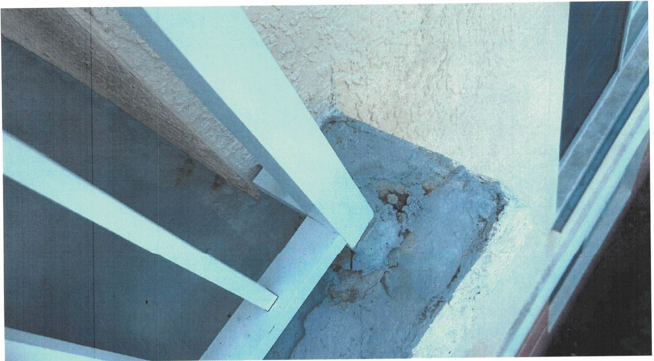
Unit 10308 - Light spalling at posts
