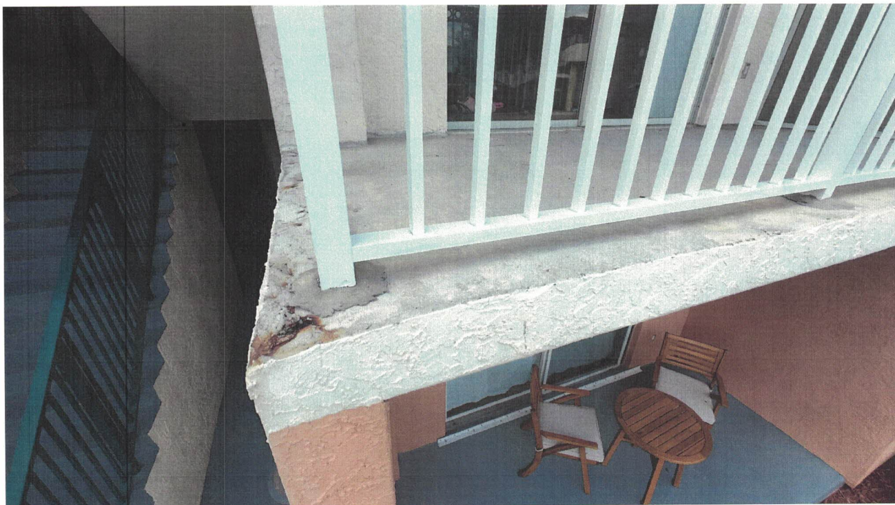
Unit 9204 - Exposed rebar
