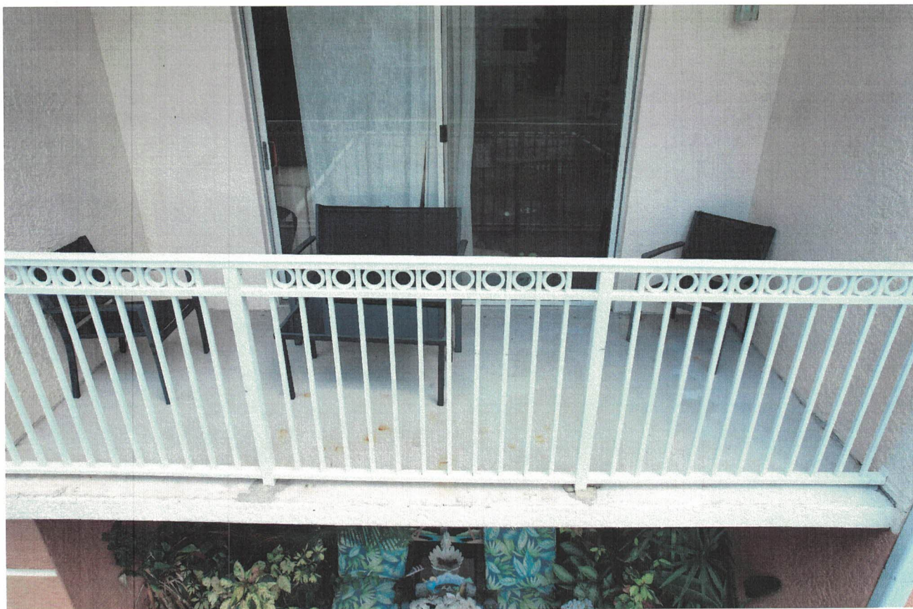
Unit 4202- Light spalling at base of posts
