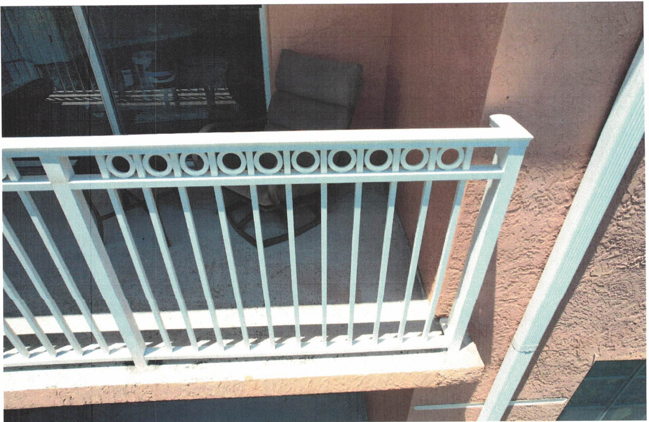
Unit 6204 - Spalling at corner post
