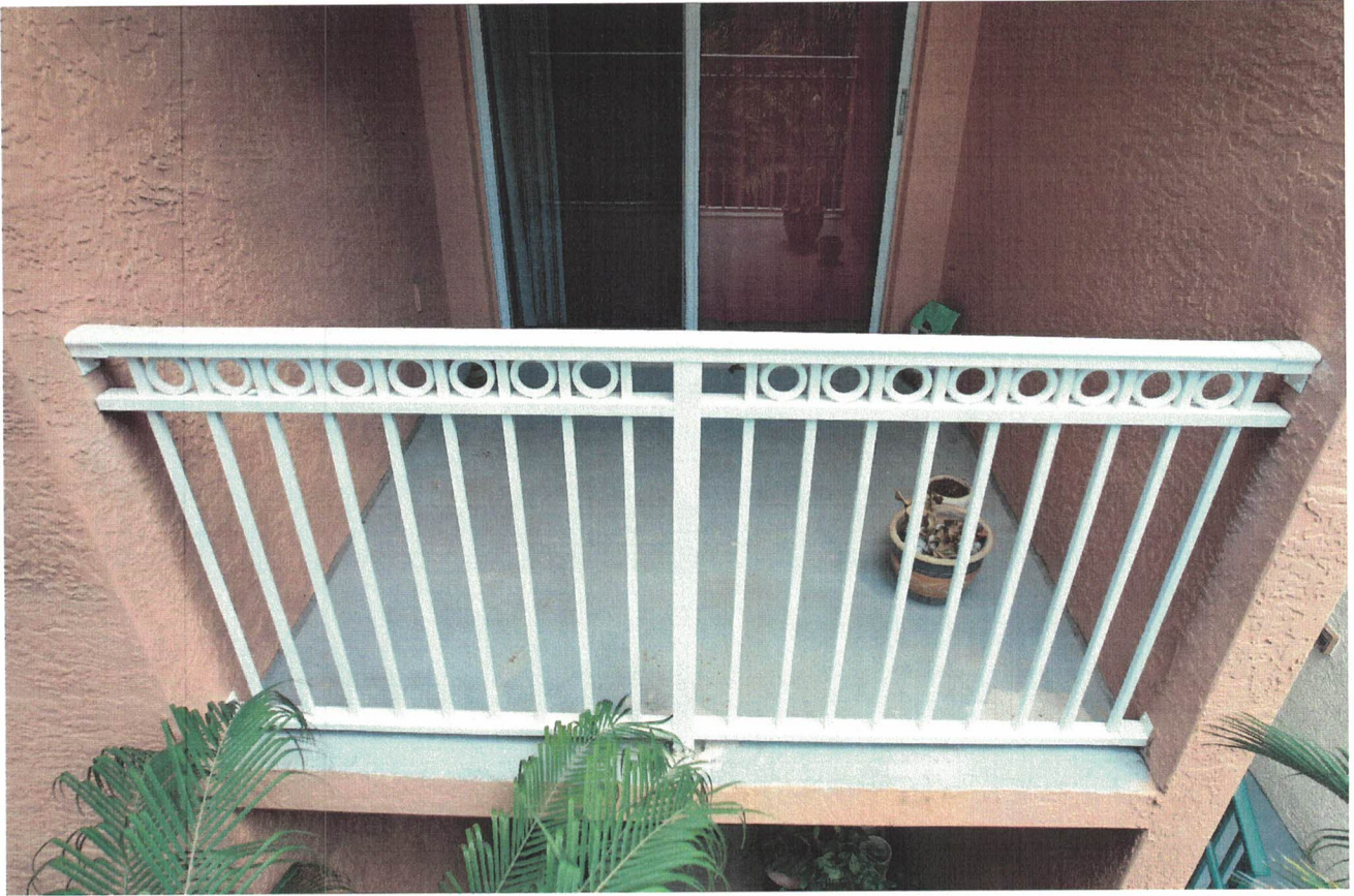
Unit 2206 - Grout missing at base of post
