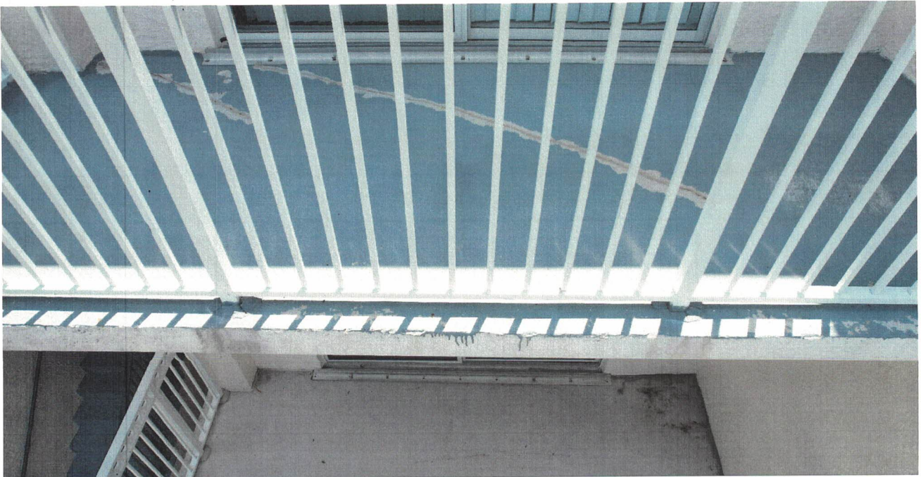
Unit 3304 - Long cracks along slab
