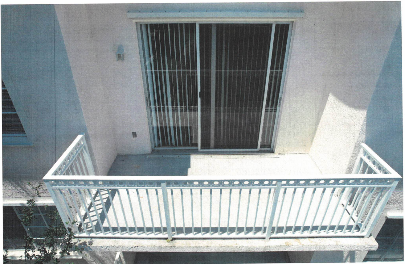
Unit 7308 - Vegetation growing out of the post socket
