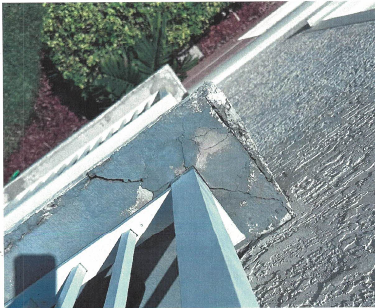
Unit 4302 - Spalling at corner post
