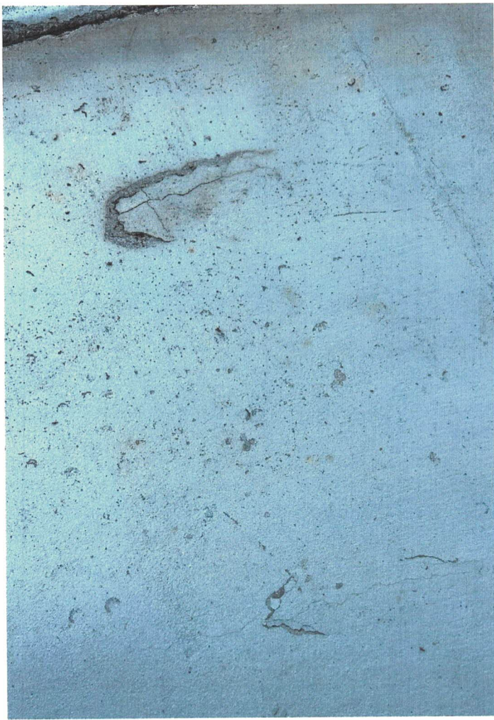
Unit 8206 - Spalling of slab / exposed rebar
