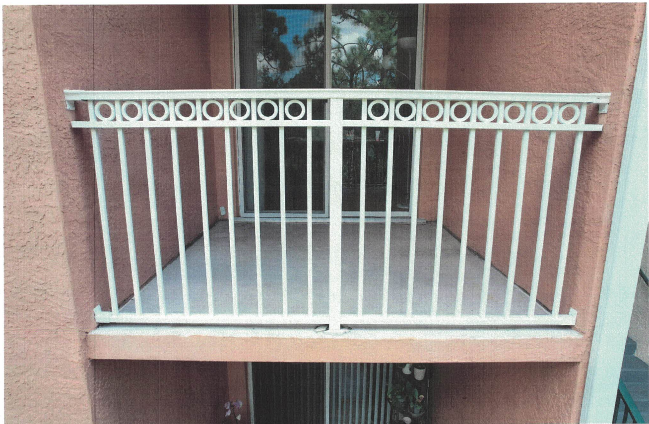
Unit 1210 - Grout spalling around base of post
